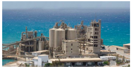
In many industrial facilities, the largest energy wasters are failed steam traps and compressed air leaks
